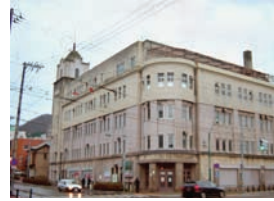
<< This hundred year old building, once a department store and city office, will be renovated for non-profit offices and community group use
