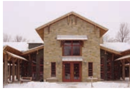
<< The Schlitz Audubon Nature Center has become a showcase for green building practices in Milwaukee
